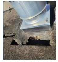
Hole in roof at Stillwater causing massive leaks
