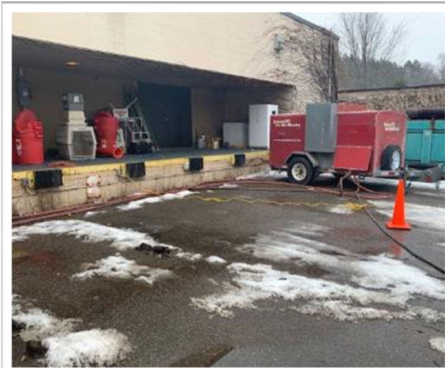
Unloading Dock serves as "ambulatory garage"
