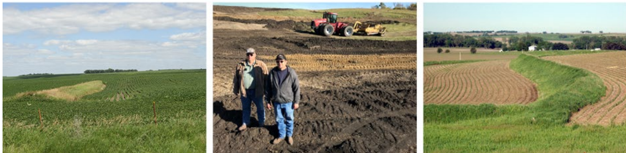
L to R: water and sediment control basin in crop field is empty in dry conditions but holds water temporarily after heavy rains; landowners pose by construction of storage basin in Pope county ag field; grass back sediment control basin slows runoff.
