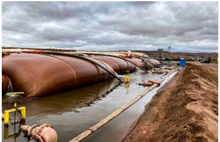
Dewatering of PCB contaminated sediment as part of the Munger Landing cleanup project in the St. Louis River Area of Concern.
