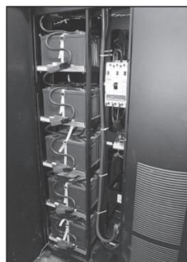
If electrical power is ever lost at the Involta data center, deep-cycle batteries — 20 to a cabinet, 80 in a bank — will provide uninterrupted service during the 22 seconds between the loss of power and when the emergency generators would begin.
