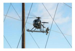
A PPL Electric Utilities employee installs a dynamic line rating sensor onto a transmission line in Pennsylvania from a helicopter. The sensors allow utilities to take into account wind speed, cloud cover and other conditions to determine if a line has more capacity. Photo Courtesy of PPL Electric Utilities.
