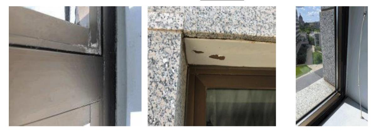
Age, Lintels Corroding, Thermal Breaks Failing, Energy Inefficient
