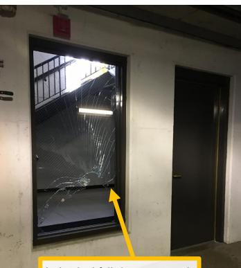
Individual fell down internal staircase (the only connection between levels of the parking ramp) and broke through window on impact. Inadequate pedestrian pathways in ramp have encouraged pedestrian use of vehicular ramp, resulting in falls and injury
