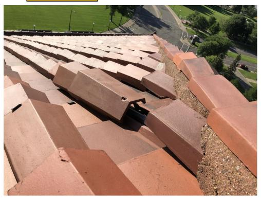
Overall Age of Roofing System, Areas of Cracked Terra Cotta Tile, Missing Nails, Leaks in Various Locations, Roof Trusses and Joists Structurally Sound
