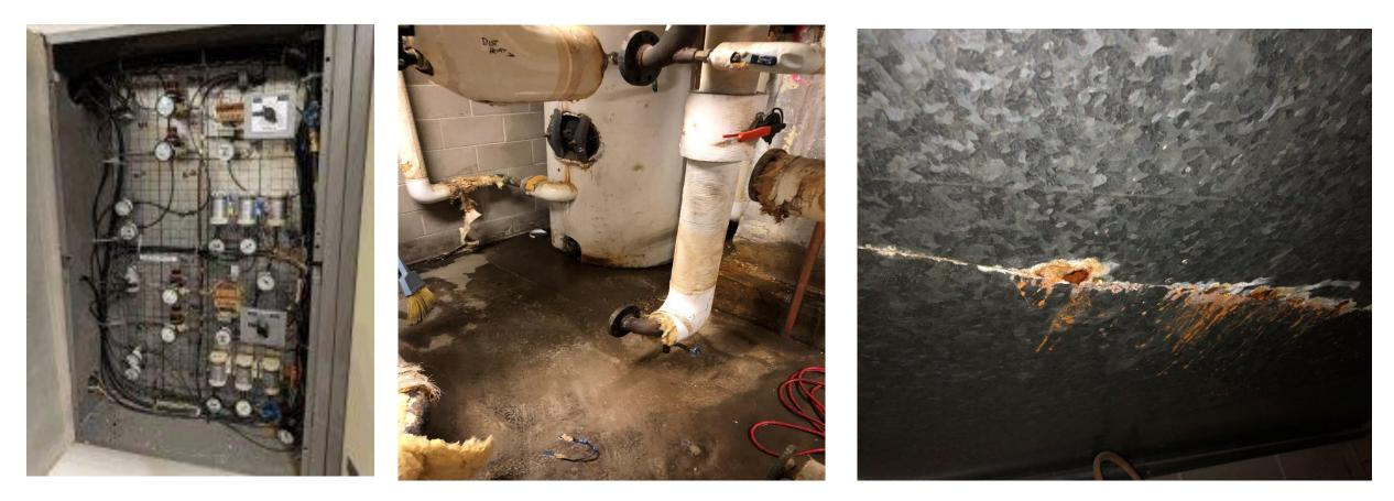
Piecemeal, Pneumatically Controlled, Pipe Connections Failing, Difficult to Maintain Constant Temps, Threat of Leaks
