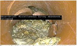
Sewer televising reports show sags, cracks, root intrusions, and several locations where the pipe is entirely collapsed.
