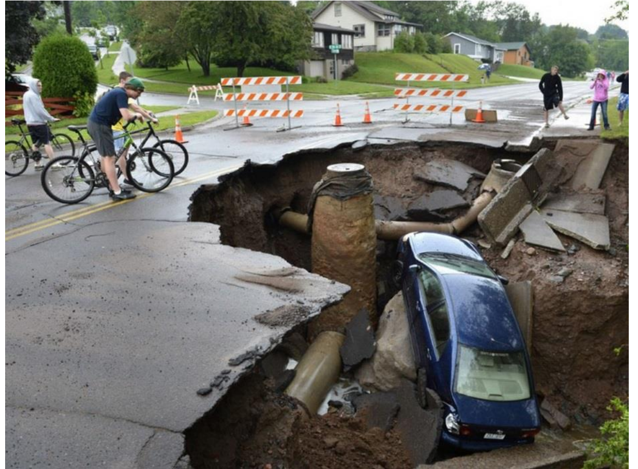
Sinkhole in Duluth caused by 2012 flooding.
